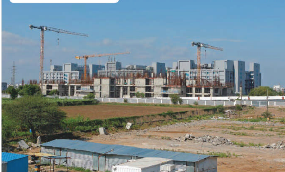
Serum's billion-dose vaccine factory, under construction
